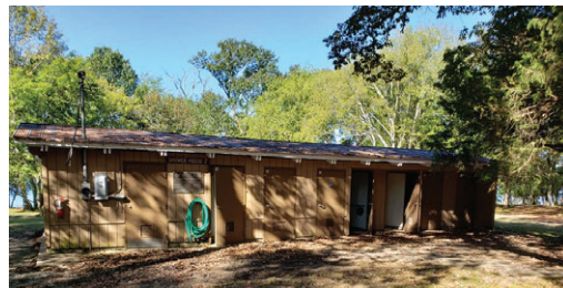
Stalman shower house before...
